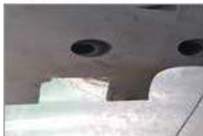
Horizontal Joint Damage
