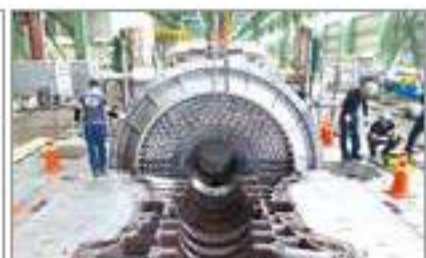
On site Maintenance & Assembly of Pressure Plate
