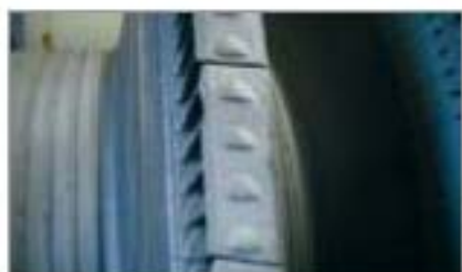
Blade Cover Damage
