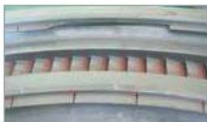
Nozzle Box Damage (Spill Strip)
