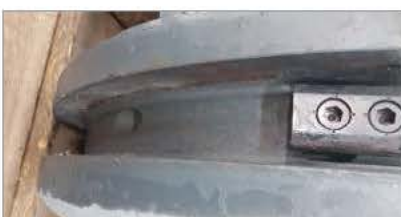
Steam Joint 손상
